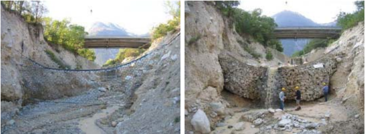
Figure 4.11. Example of flexible ring-net debris-flow barrier before (left) and after (right) debris-flow event (Figure 3; Wendeler et al., 2008b).
