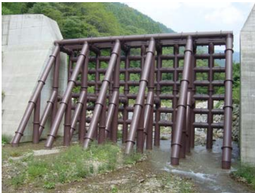
Figure 4.8. Concrete and steel pipe sabo dam. (Photo 4; Mizuyama [No 1], 2008).
