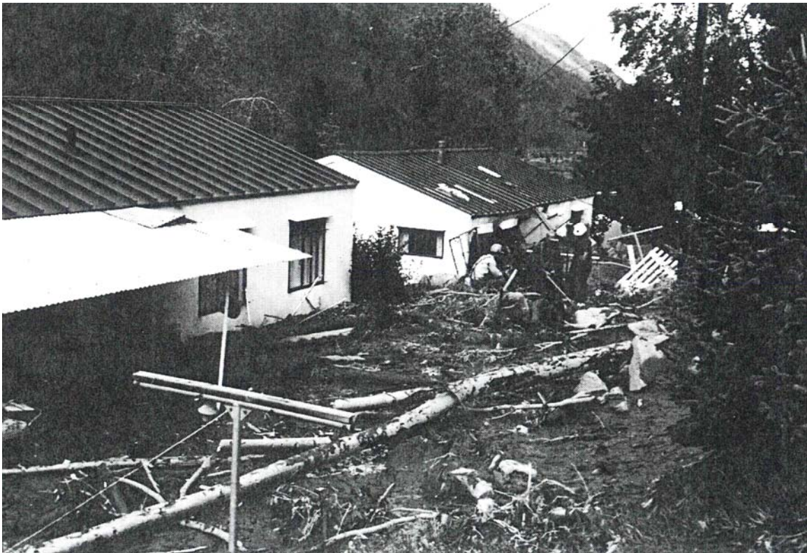
Figure 4.2. Historic photograph taken within Town of Telluride showing debris and damage caused by 1969 debris flow event.
