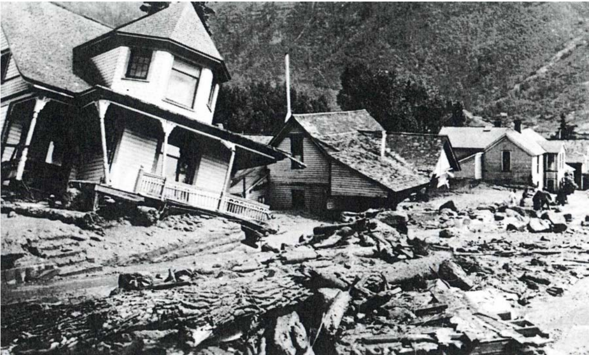
Figure 4.1. Historic photograph taken within Town of Telluride showing debris and damage caused by 1914 debris flow event.
